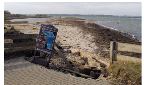
The damages to tourist infrastructure caused by coastal erosion, as seen here in Laboe, pose great challenges to these communities.
