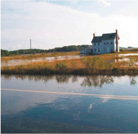
The yard surrounding a house in Dorchester County, Maryland is flooded during a spring high tide.
